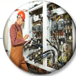
BMS / Energy Management
